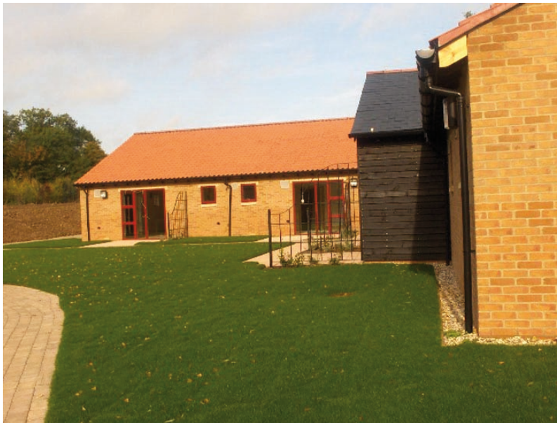
Picture 5: View of New Farleigh Hospice ward section (under construction)
